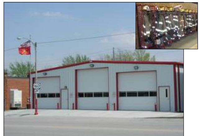
Community Facility Direct Loan & Grant Program funds were used to build this Fire Station in Moline, which replaced a previous facility that did not have enough space for the Department's trucks and equipment.
