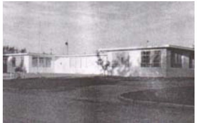
The first Starkey School, after completion in 1952.
